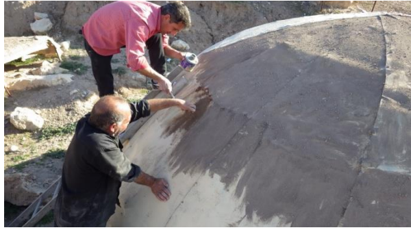
Fig. 5: Covering half the dome with dirt (5a, on the left) and the experiment with burlap (5b, on the right)
