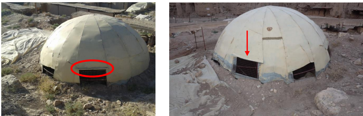
Fig. 4: Showing the openings and the drains above the openings
