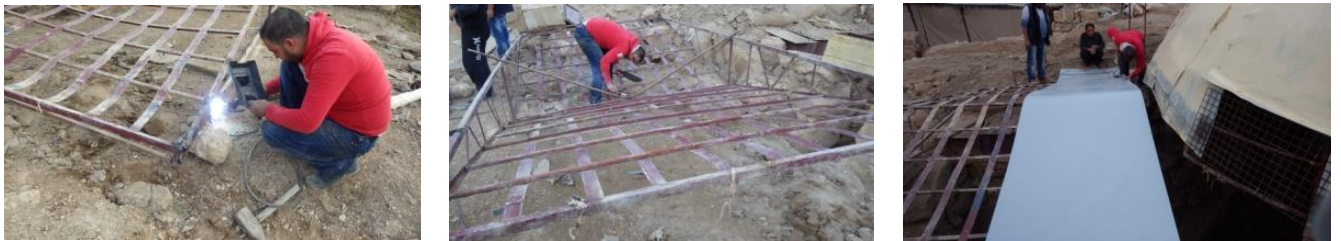
Fig 7: Different stages of work on the entrance
