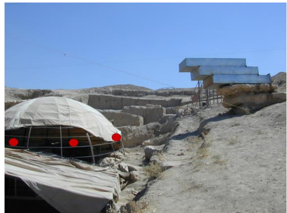
Fig. 1: Photos with the indication of the openings to be created in the new metal dome for aeration and light inside the abi
