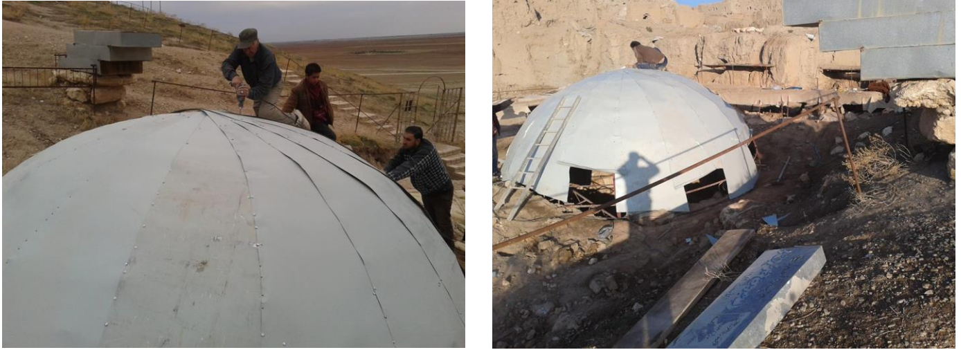
Fig. 3: Sabah Khasseem at work (left) and detail of the openings at the base of the new abi dome
