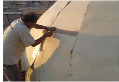
Fig. 5: Covering half the dome with dirt (5a, on the left) and the experiment with burlap (5b, on the right)
